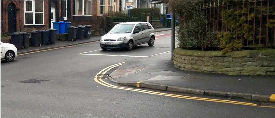
Although the proposals include for relocation of this crossing, the provision of the full-height replacement kerb face would still leave an excessive footway gradient falling towards the carriageway.
