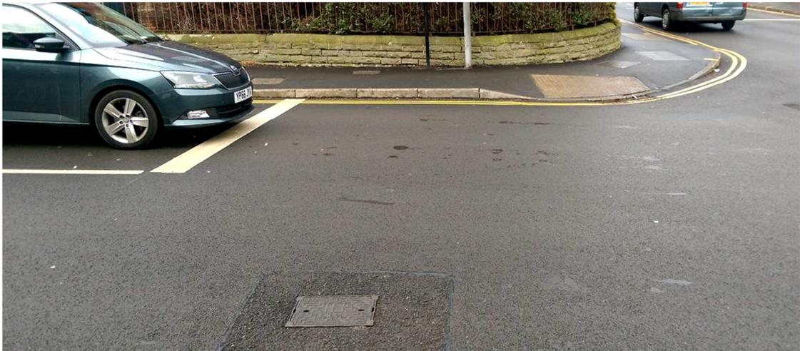
The ironwork cover is worn and polished, and there would be a likelihood of pedestrians slipping, falling and sustaining injury if stepping on the cover, particularly during or after inclement weather conditions.
